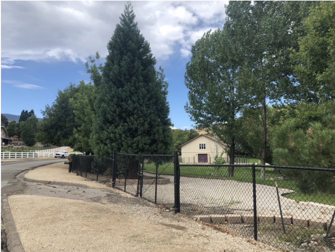
Southeast View of the Existing Barn
